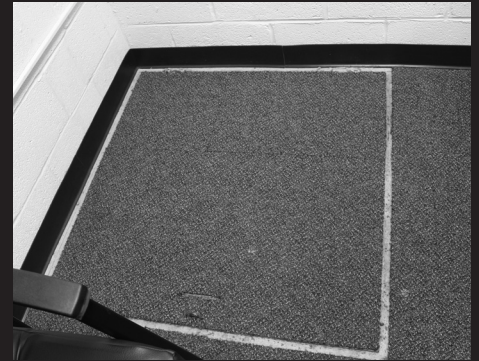
The second entrance, a trap door. It was locked and has not been opened since renovations, so we could not get inside.
