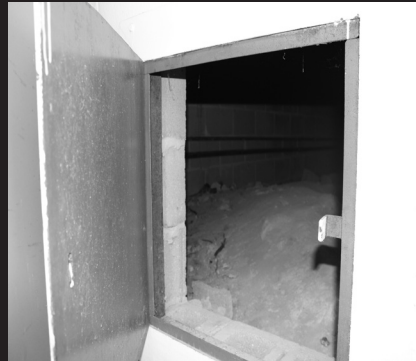
The otherside of the door. The floor of the tunnel is dirt and there is no lighting.
