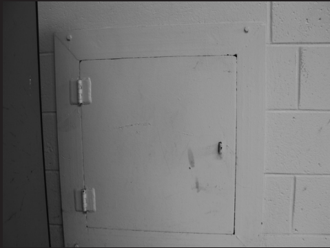
This door, found in a wall in the school, is an entrance to a tunnel under a staircase.
